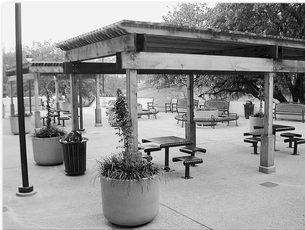
View of the newly redesigned south plaza of Welch Hall looking toward Inner Campus Drive. The new plaza, recently resurfaced to stop rainwater leaks into classrooms below, has become a popular venue for relaxation, study, dining and even outdoor class sessions on sunny fall days.
