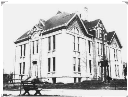
The Chemical Laboratory, home of the Chemistry Department from 1892 to 1926. It stood near where the Biology Greenhouse is today.
